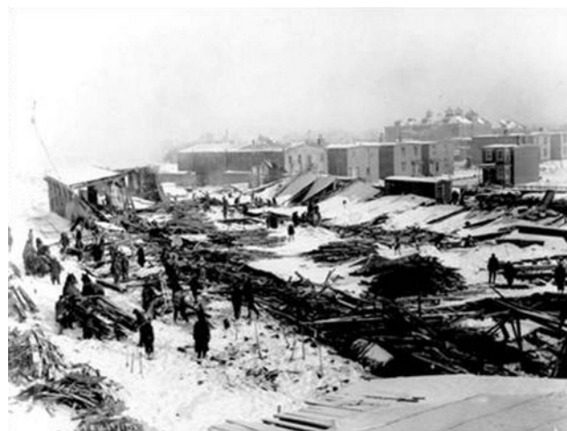
Figure 2 Collapsed buildings in the North End of Halifax, Nova Scotia, Canada. Printed with permission from PANS, Charles Vaughan collection, N-7036.
